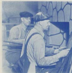
Al Moore and Earl Unroe, Maintenance Department carpenters, are shown above as they prepared the fireplace through which Santa Claus came to our party.
